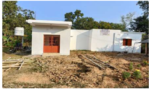
Construction of Multipurpose Community Centre
